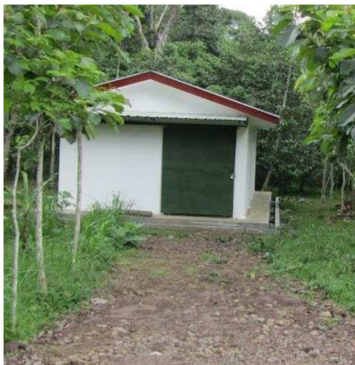
New feedmill building
